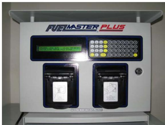
MoDOT's new statewide automated fuel management system will help the department gain efficiencies and account for petroleum products by providing the ability to track fuel deliveries, fuel dispensed per transaction and site inventory levels.
