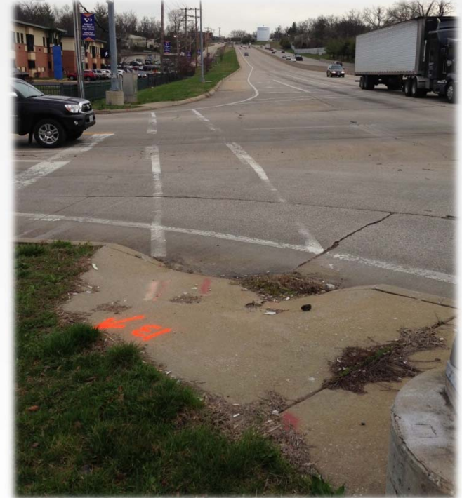
SW Corner Looking North Toward VP Schools
