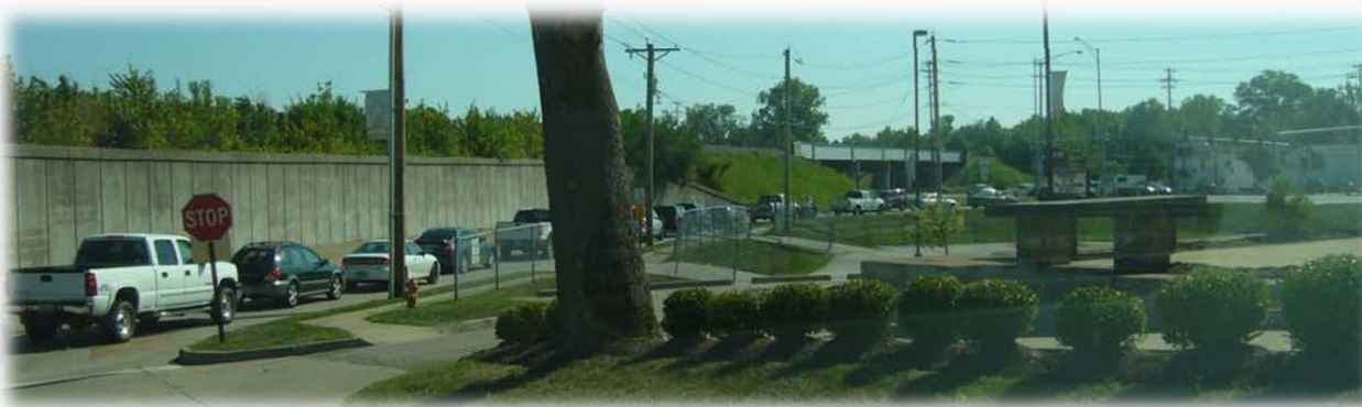
Forest Ave at Route 141 Looking West – PM Peak
