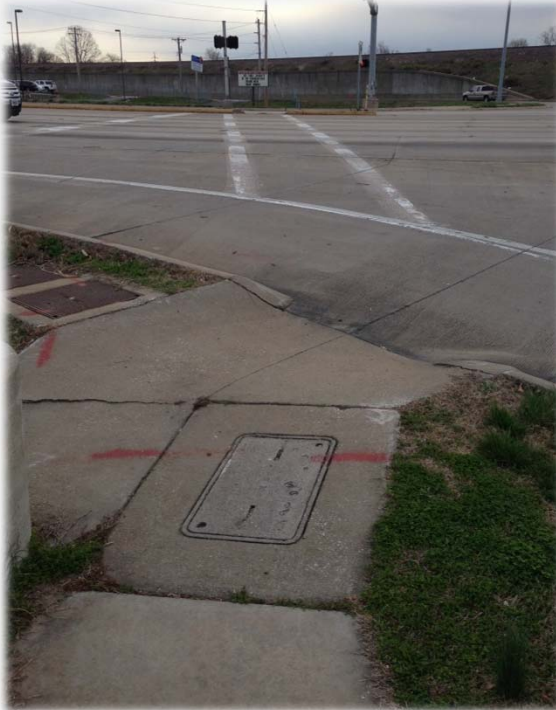
NW Corner Looking East
