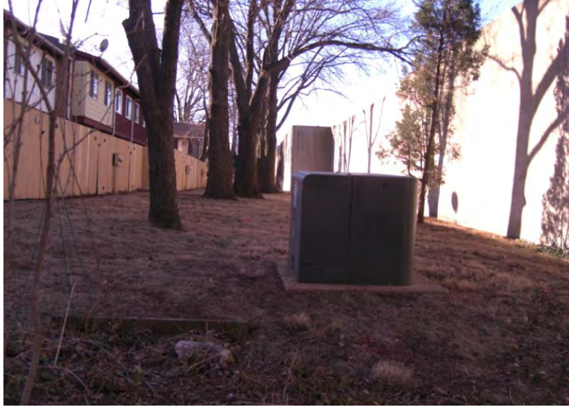
Existing Noise Barrier between I-170 and Granada Condominiums
