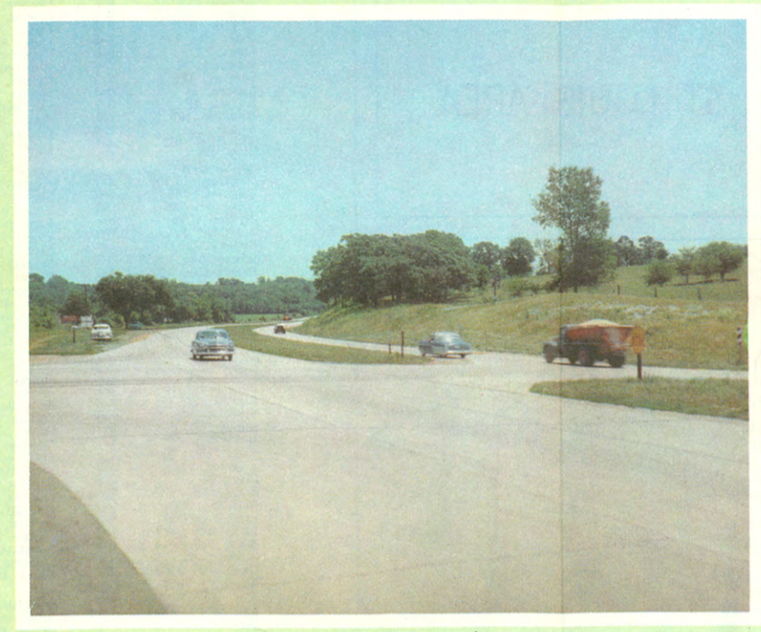
US Route 40 at Route 0, Jackson County
