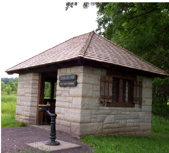
This bus shelter at the Shaw Nature Reserve in St. Louis was built by the Civilian Conservation Corps (CCC) in 1939 and relocated here in 2002.
