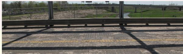
The superstructure carries the deck whose function is to transfer live loads and dead loads off the deck to other bridge components.
