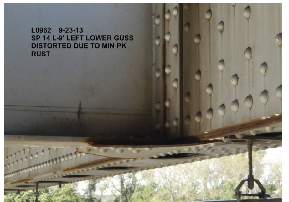
Pictures of Rocheport Bridge's condition, illustrating need for replacement. Source: MoDOT
