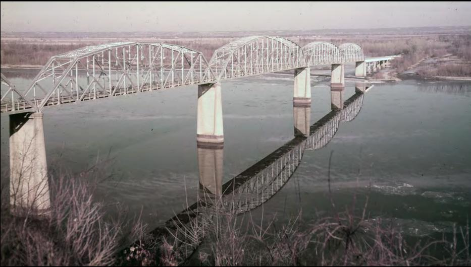
The Champ Clark Bridge is a 5-span, Pennsylvania through truss with 6 steel plate deck girder approach spans on the East end. It was built between 1926 and 1928 for the Missouri-Illinois Bridge Company and cost \$1,000,000 to construct. It opened on May 15, 1928 and operated as a toll bridge until 1952, when it was freed.
