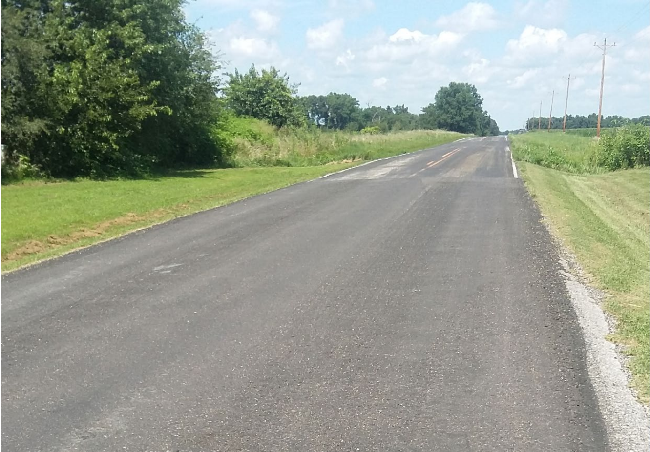
Typical asphalt pavement repair
