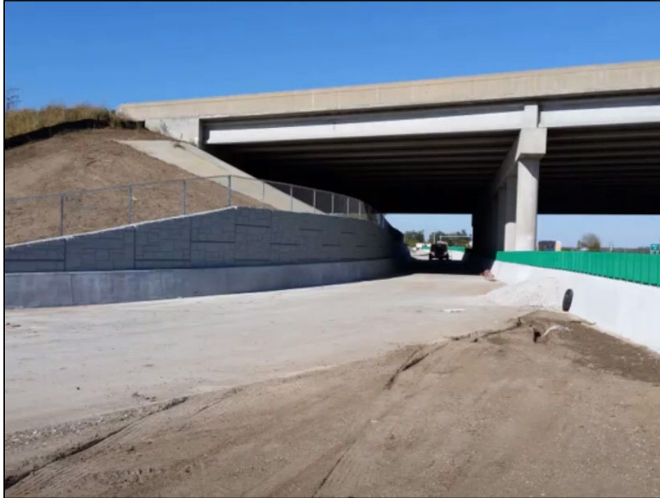
CFA Tangent Retaining Wall
