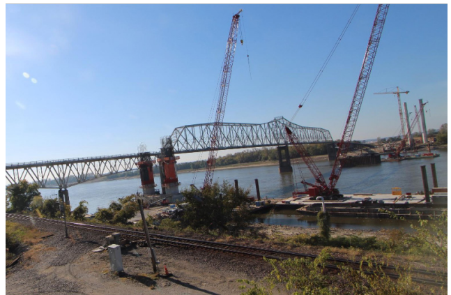
Construction continues on the new Don Welge Memorial Bridge.
