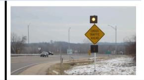
Flashing Beacon on Advance Warning Signs Adds flashing lights onto existing advanced warning signs for added visibility of the sign.
